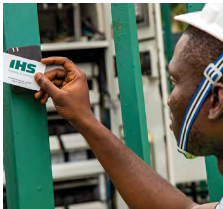
Running safe, secure tower sites.
